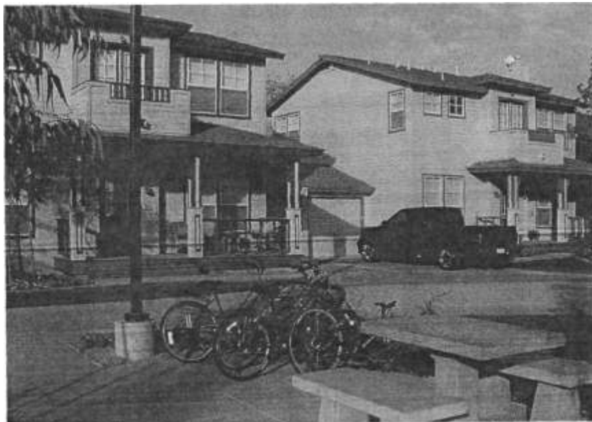
Figure 11.9 These multifamily homes in an infill development of Tempe, Arizona reduce outward sprawl and encourage alternate modes of transportation, as the built-in bike racks indicate. The front porches add a New Urbanist touch.
